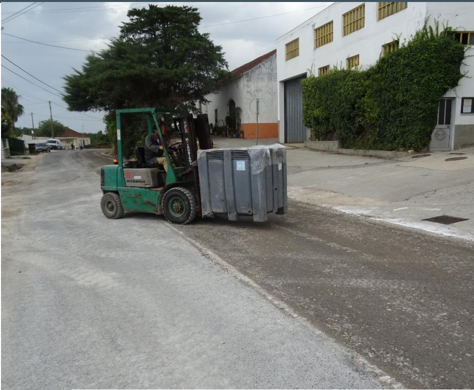
Minimum disruption to local business, Fork Lift crossing Recycled Lane after 30mins, NO damage
