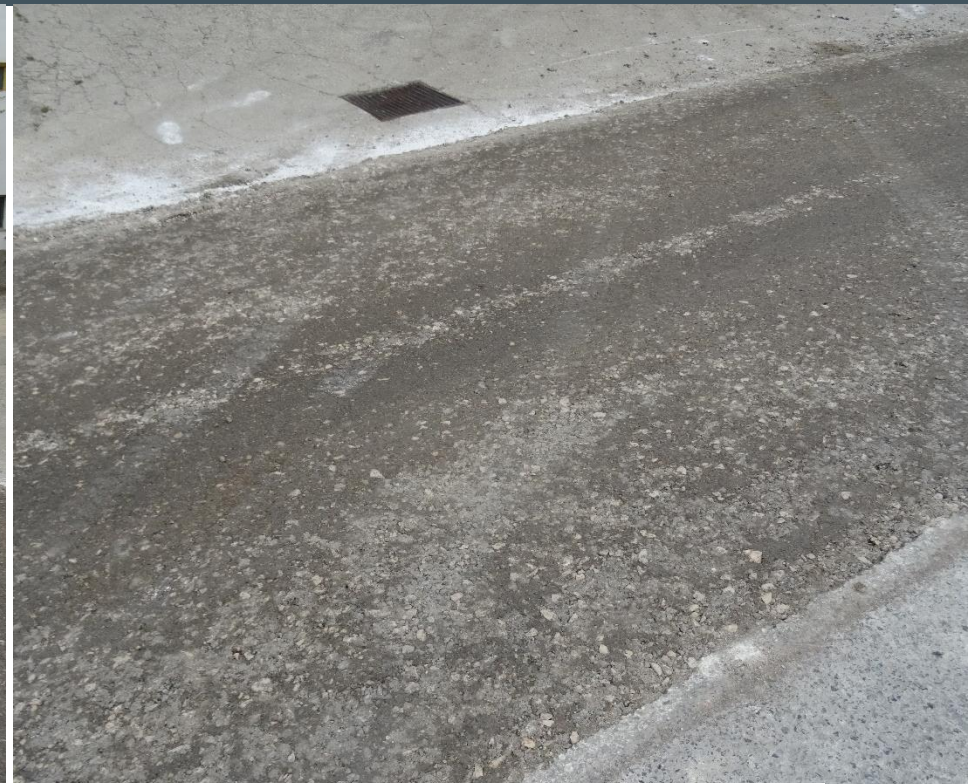
Minimum disruption to local business, Fork Lift crossing Recycled Lane after 30mins, NO damage
