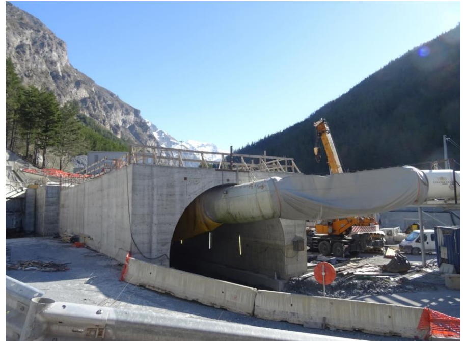
Frejus Tunnel during construction
