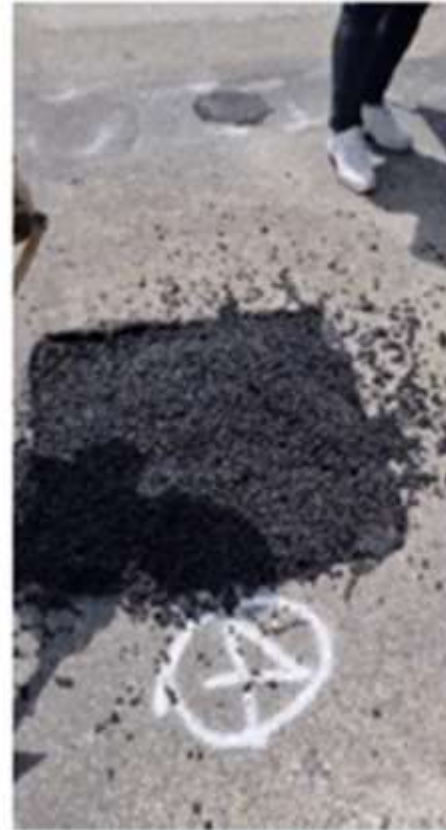
4. Applying of the mixture
