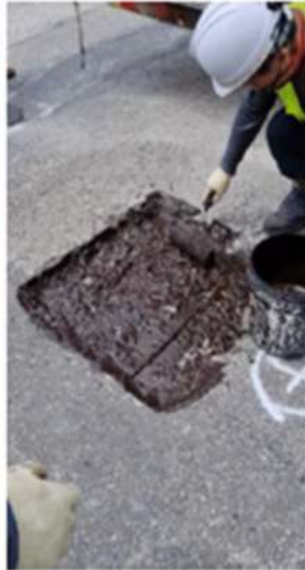
3. Primer coating application
