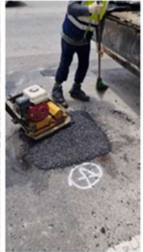
5. Compaction of laying surface
