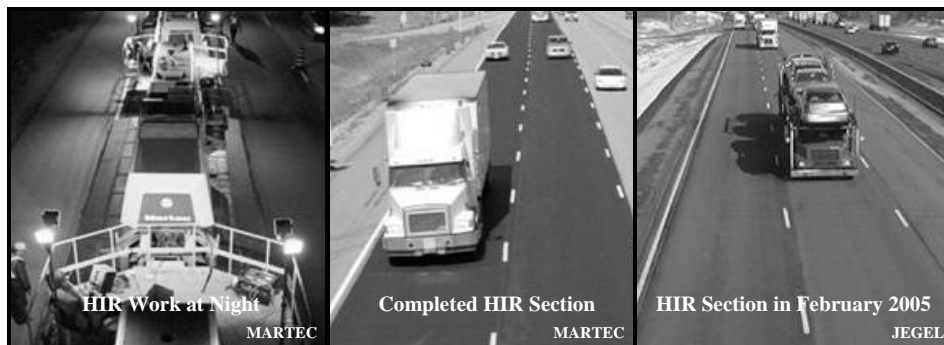
Photograph 4 Ontario Highway 401 September 1999 Hot In-Place Recycling (HIR) Demonstration Project, as Part of Five Rehabilitation Strategies Comparison
